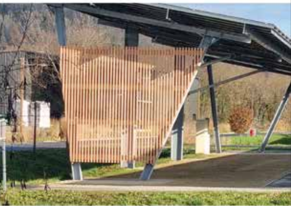
Bardage ombrière VDD & See You Sun 38110 Saint Clair de la Tour
